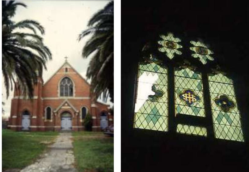
Fig. 10: Exterior of 1913 Holy Trinity Anglican Church, Port Melbourne in 1997
