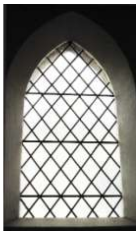
Fig 1: Original leadlight in Holy Trinity Church (formerly the church hall)
